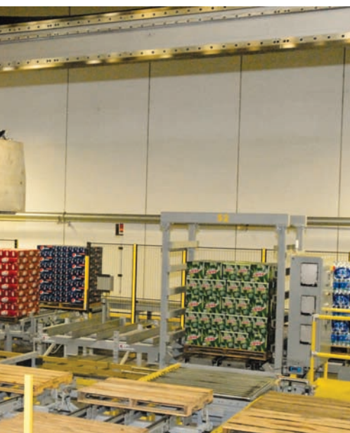
Layer picking via gantry robots
