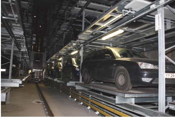
Figure 3: Below ground: Insight into Copenhagen's second fully-automated parking garage.
